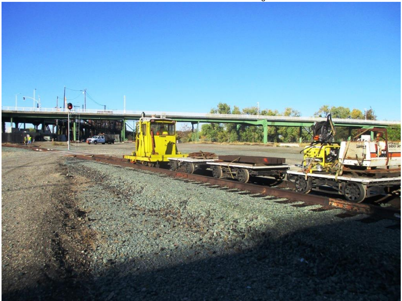
Ready to roll: with no impediments, the MOW Team work-train waits (and waits, and waits) for a green light
