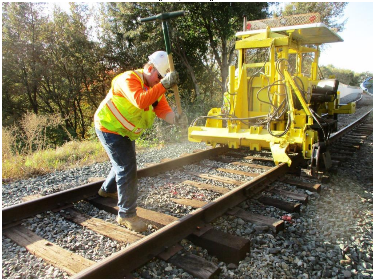
Chris H. drives the last spike. With that, principle construction on the Zoo Line is complete!
