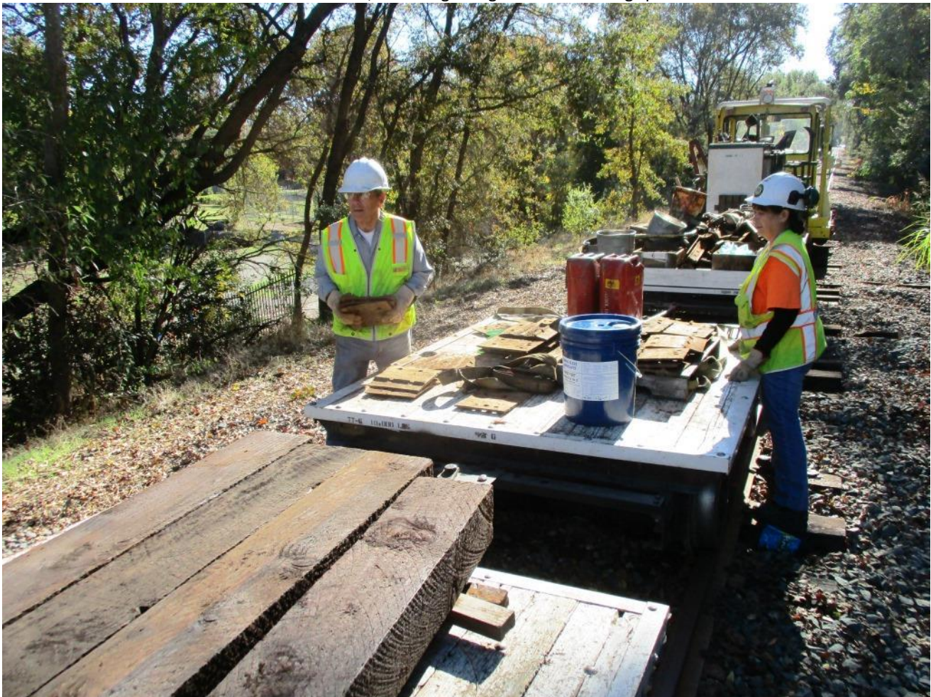
Mike T. and Pam distribute tie-plates to needy ties
