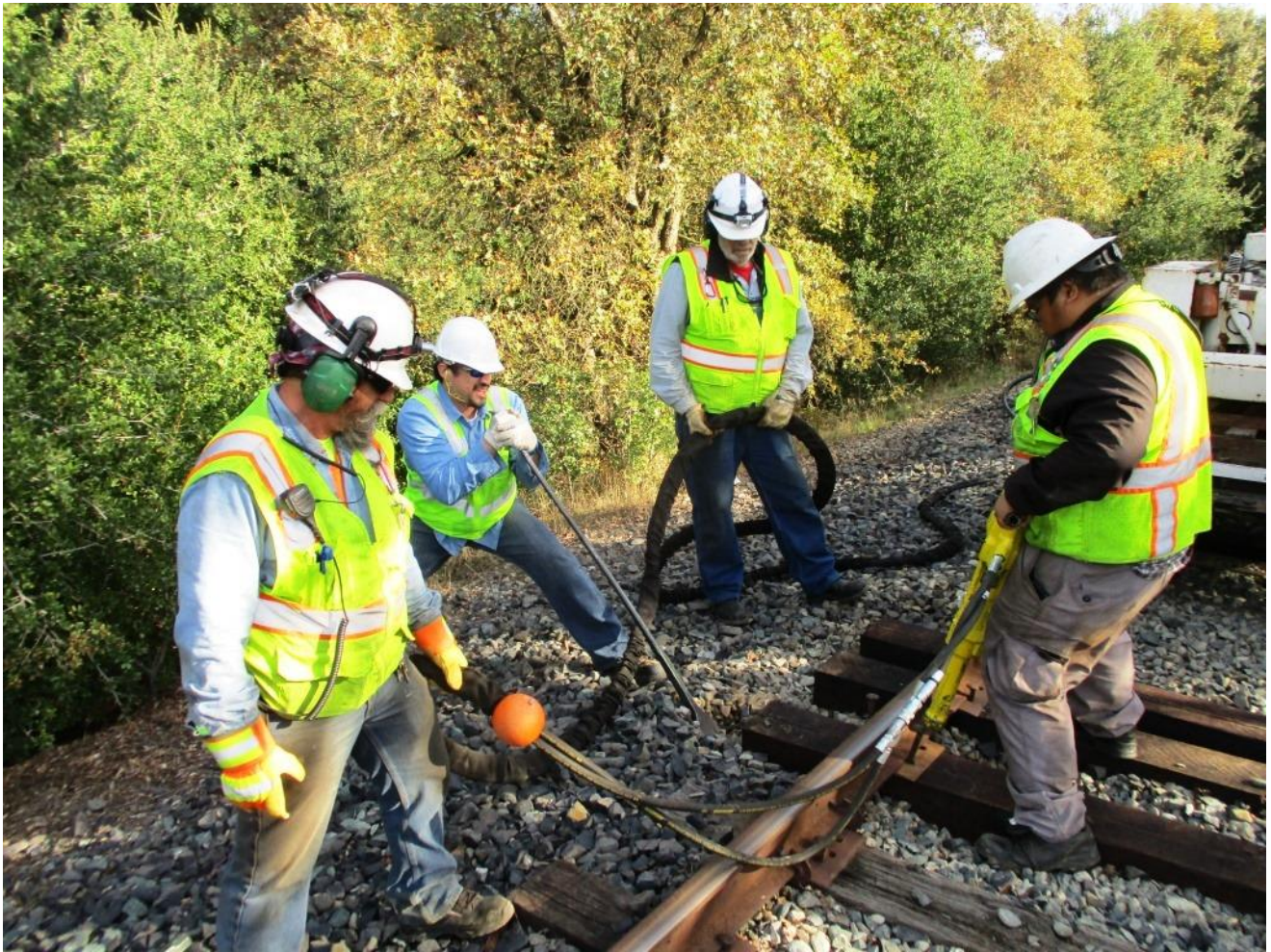
Jose nips-up the tie as Anthony drives the spike. Joe and Art guide the hydraulic hoses
