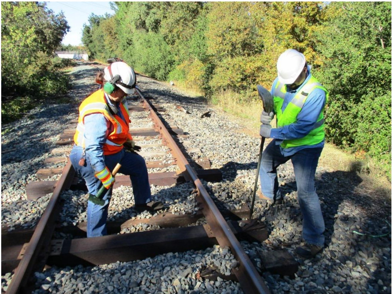
Jose uses the narrow-end of the nipping-bar to nip-up a tie as Heather comes in to set spikes in it
