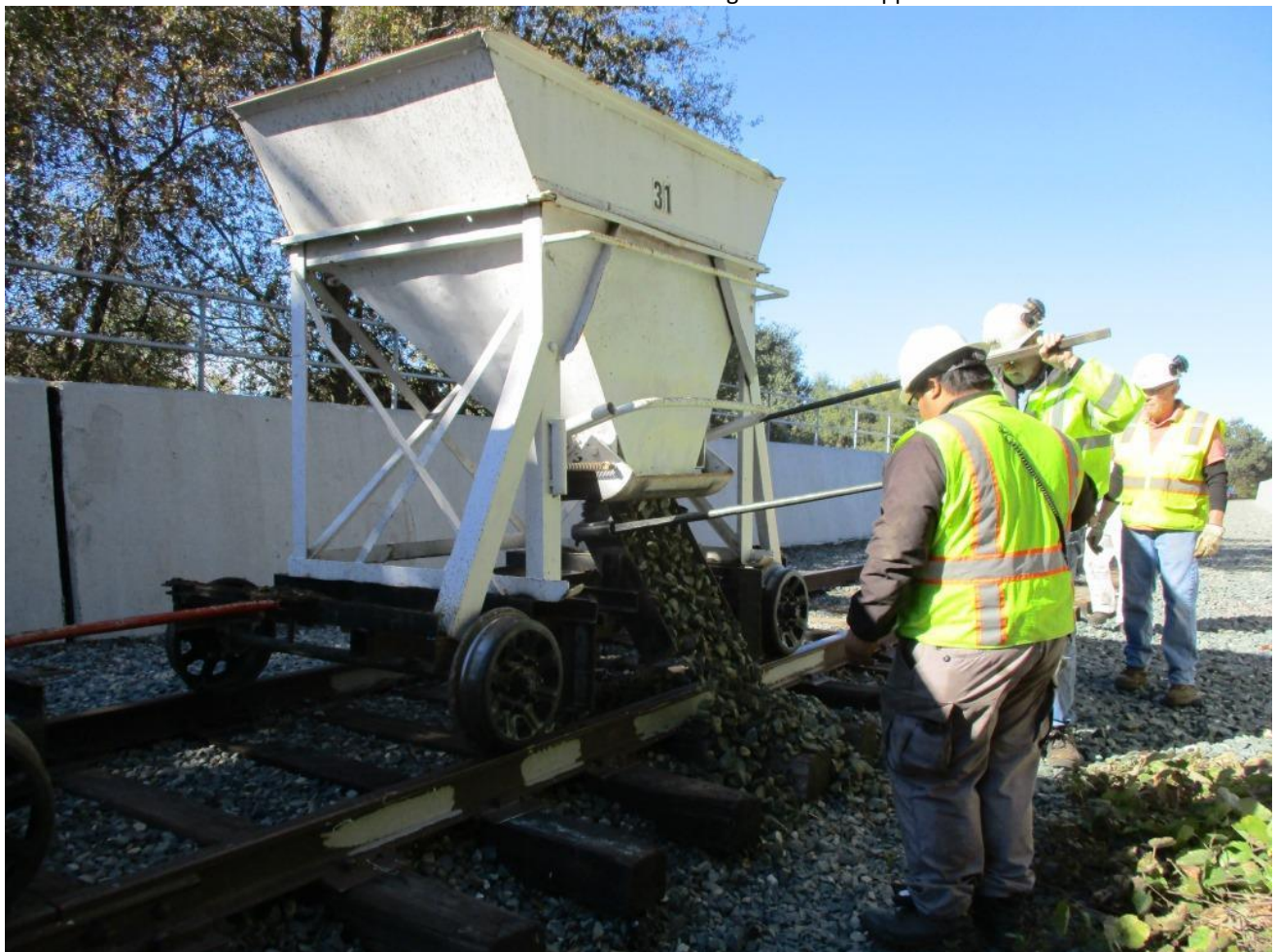
Anthony and Alan discharge rock from the side-dump car to fill in an undercut area
