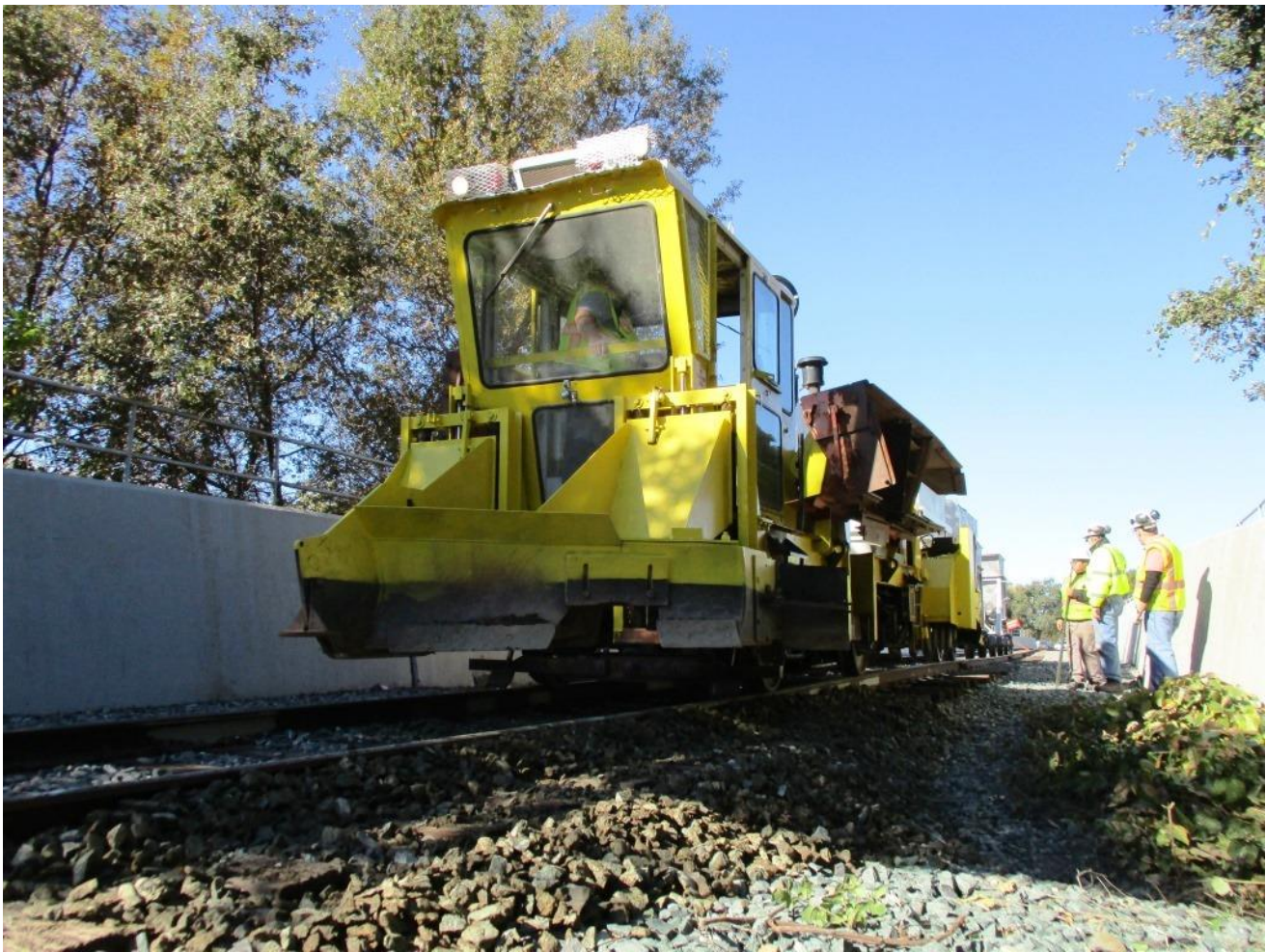
Chris C. arrives on site with the ballast regulator and hopper cars
