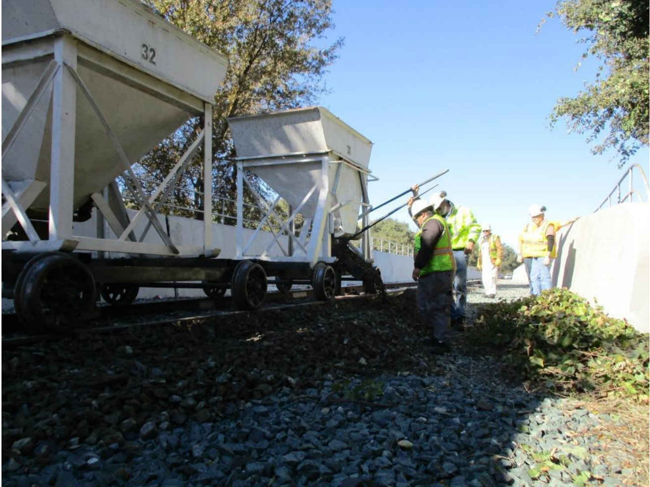
Anthony and Alan make another pass over the area being filled-in
