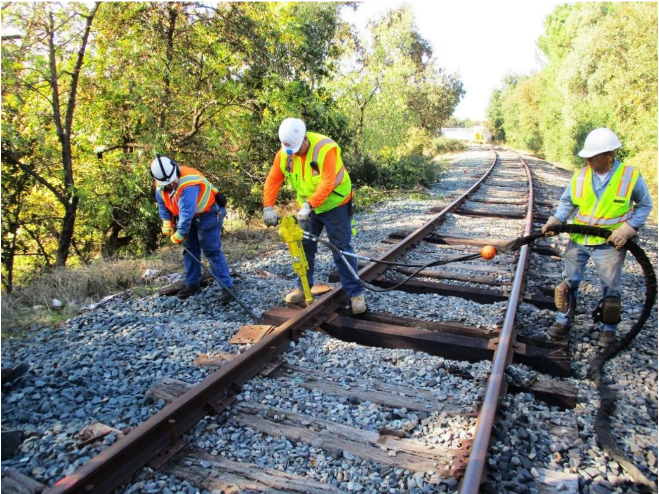
Heather nips-up the tie as Chris H. drives spikes with the hydraulic spike-driver while Mike T. guides the hydraulic hoses
