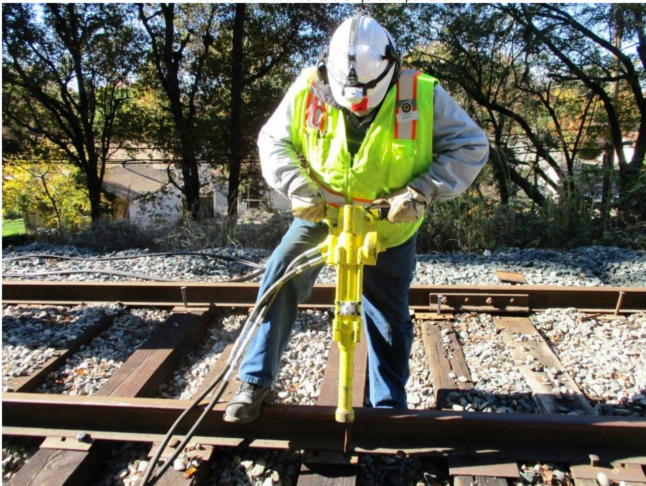
Art was first-up with the hydraulic spike-driver
