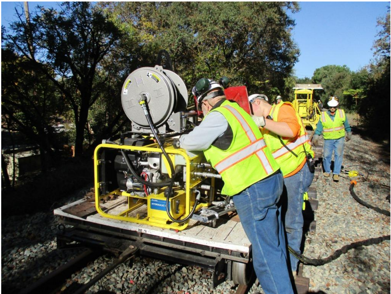
Art and Chris H. add fuel to the hydraulic power unit
