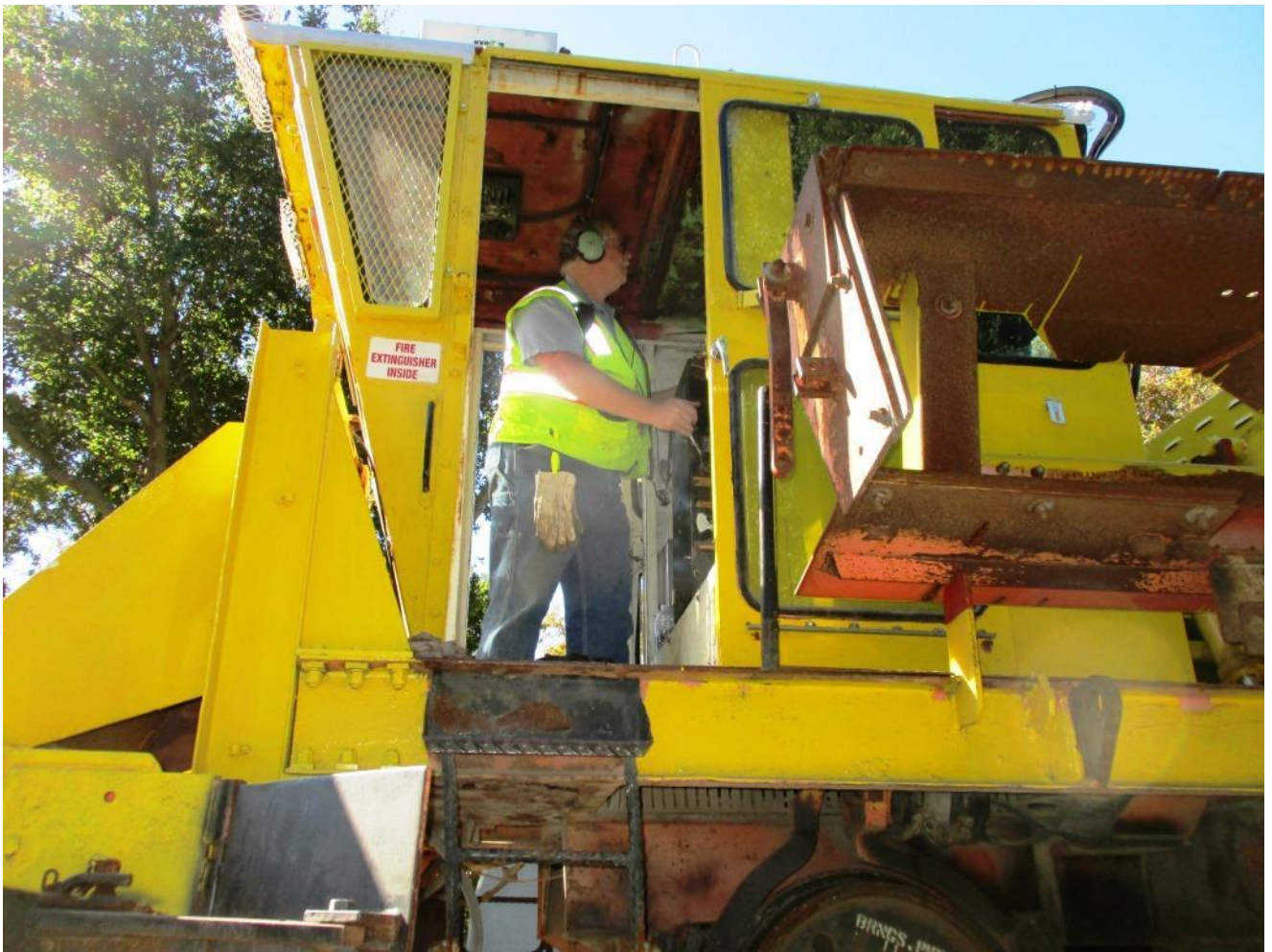
Chris C. keeps a close eye on the ballasting operation as he slowly pulls the rock-cars south
