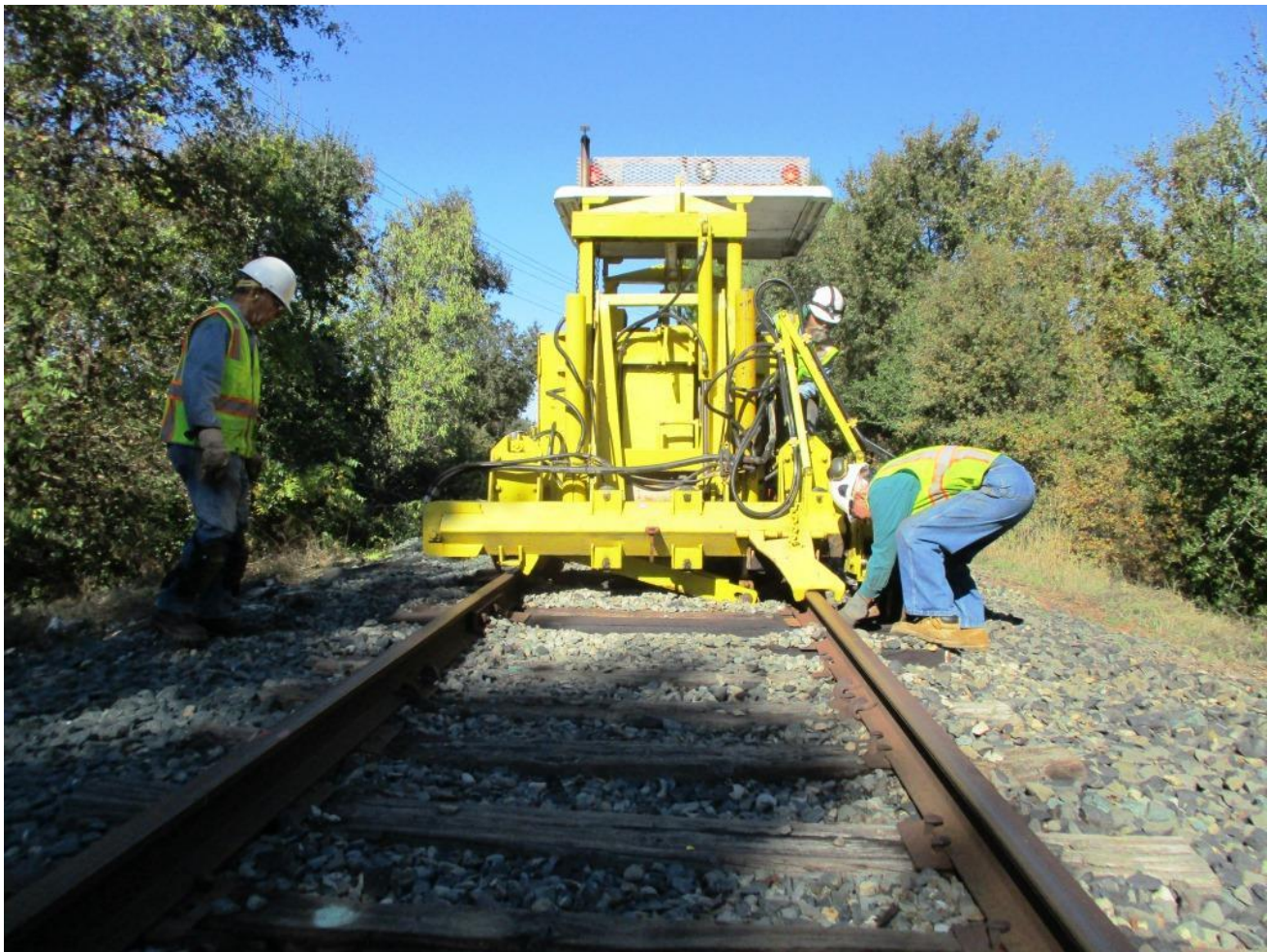
Joe uses the Jackson 125's track-lifting ability to allow Clem and Mike T. insert tie-plates with ease
