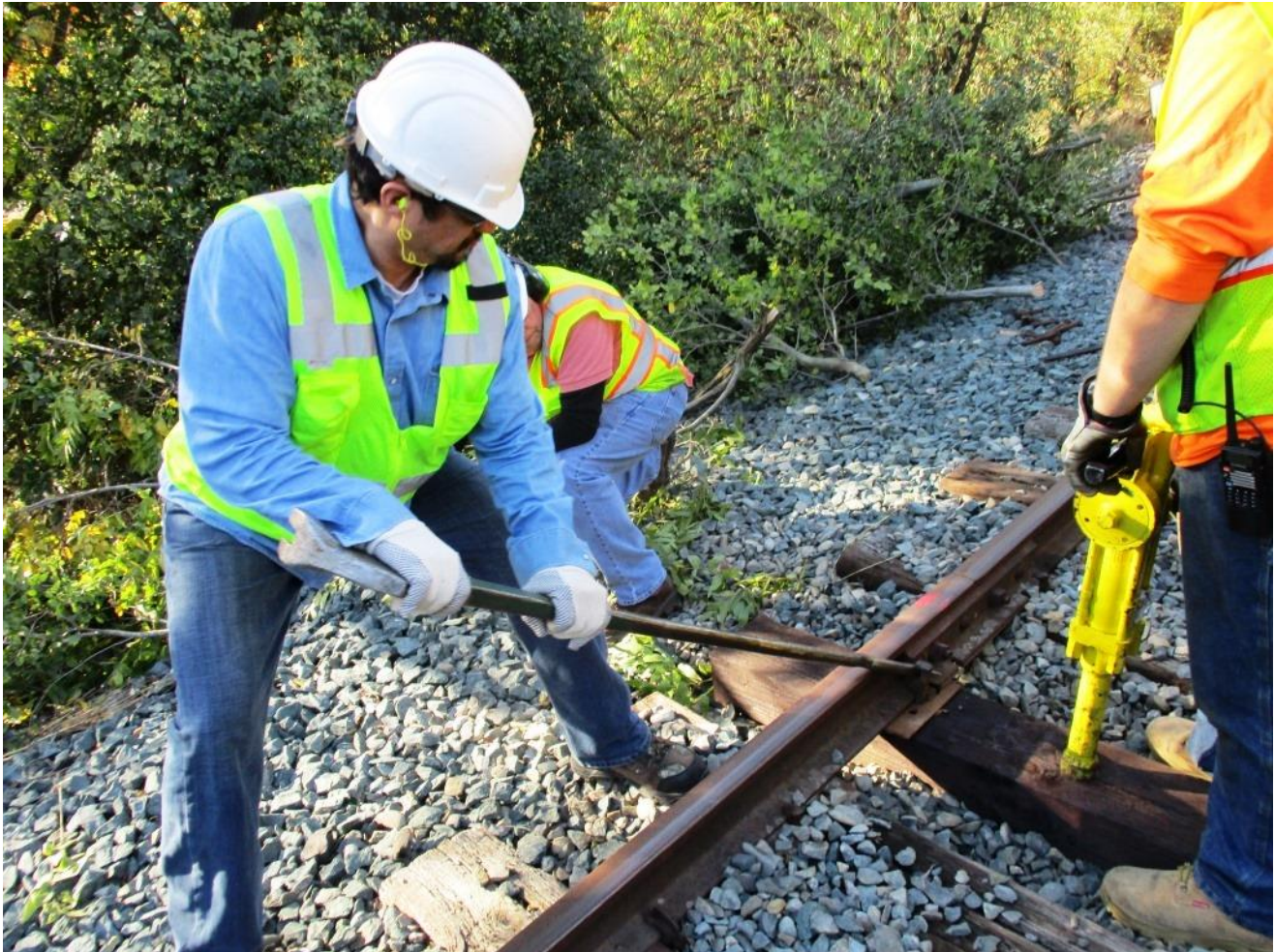
Jose uses the leverage from a claw-bar to unbend a bent spike
