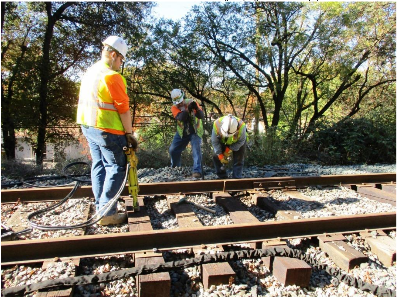
Chris H. is next up on the hydraulic spiker as Joe sets a spike and Mike F. nips-up the tie
