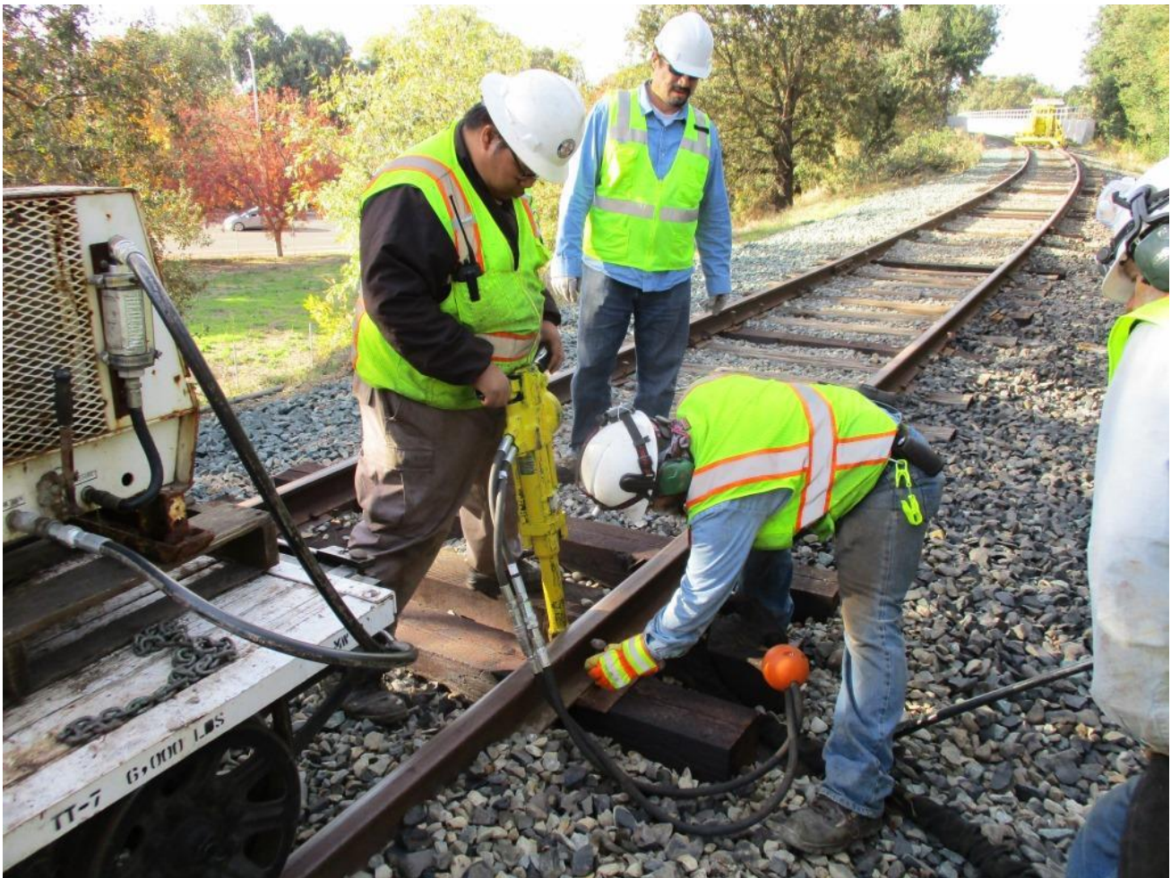
The spike-driving craziness is spreading! Now Anthony's caught it. Meanwhile Joe sets a spike
