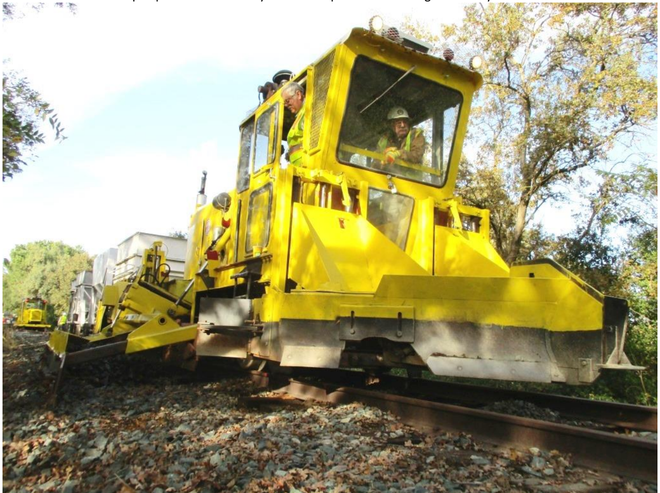
Chris C. and Mike H. deploy the regulator's wing to pull rock alongside the track and fill in some of the holes
