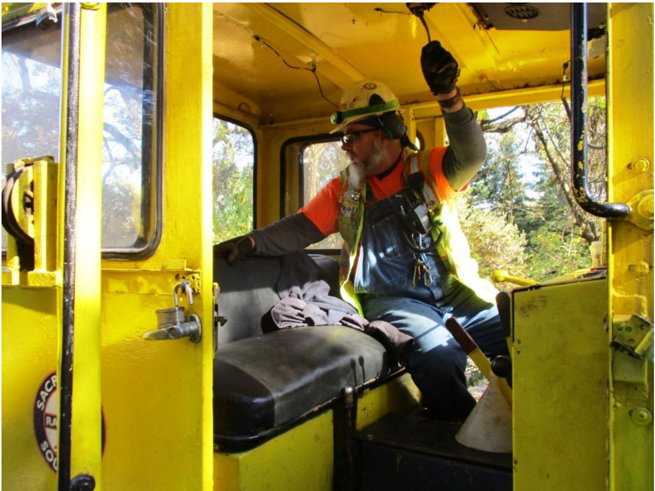
Mike F. slowly shoves the track machines following the progress of the crazy spikers
